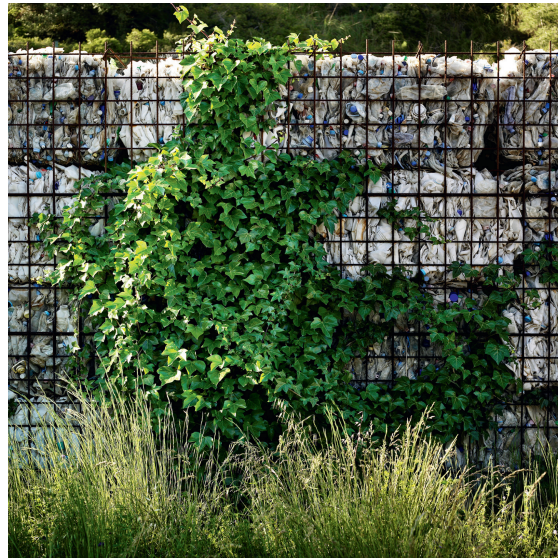
Figure 16.3.10 Detail of plant walls, built of nondegradable products of the old landfill (Sánchez Fabra, 2015).
